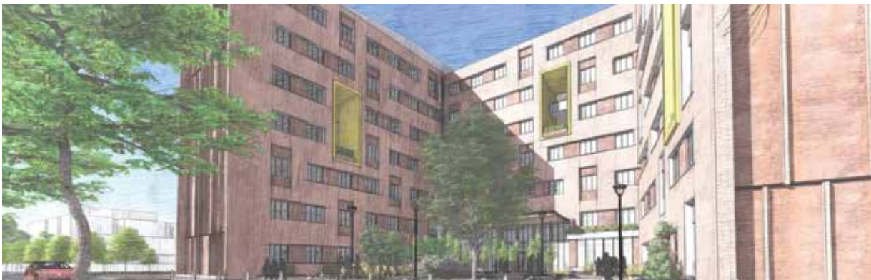
The new hostel building will be able to accommodate around 500 female students on campus
